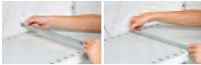
Assembling the guide rails for multibox
