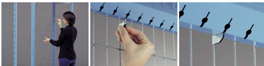
Assembling the mesh panel
